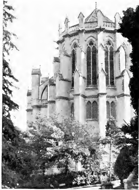
"THE FINEST VIEW IS THAT OF THE APSE."— MONTPELLIER.
